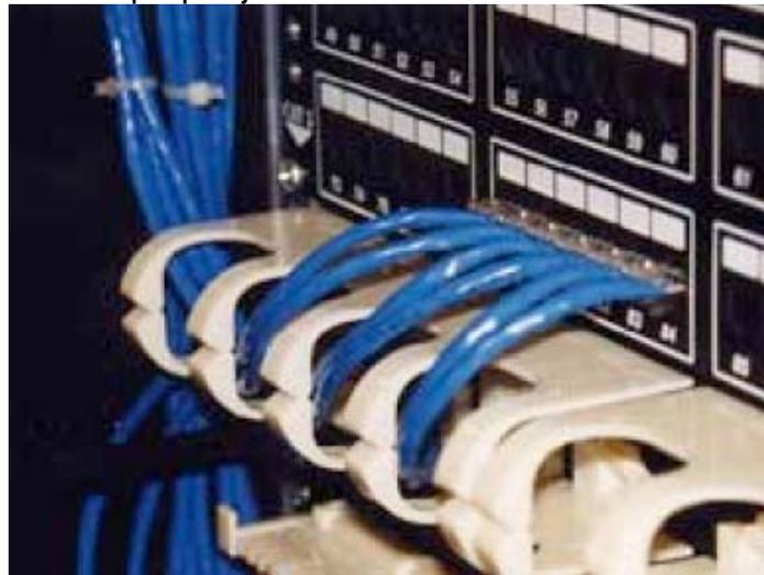
Patch panels can have massive number of cables, so managing these cables can be quite a task in itself. It is important to keep all cables neatly bundled and labeled so they can be moved when necessary. However, it is also important to maintain the integrity of the cables, preventing kinking or bending in too small a radius which may adversely affect frequency performance.
