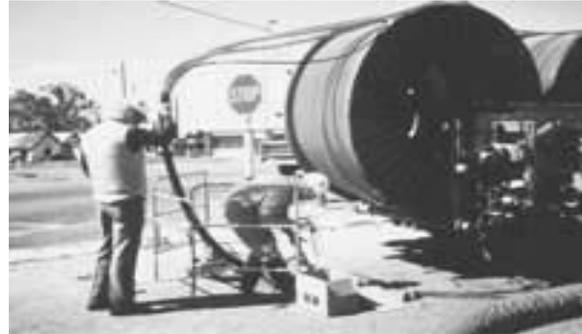
Long distances mean cables are spliced together, since cables are not longer than about 4 km (2.5 miles), and most splices are by fusion splicing. Connectors (SC, ST or FC styles) on factory made pigtailed cables are spliced onto the end of the cable. After installation, every fiber and every splice is tested with an OTDR.
